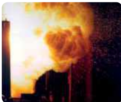
Switchgear explosion due to arc fault
