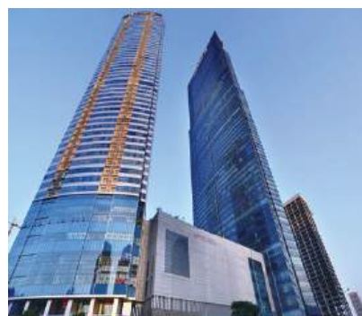
Keangnam Hanoi Landmark Tower
